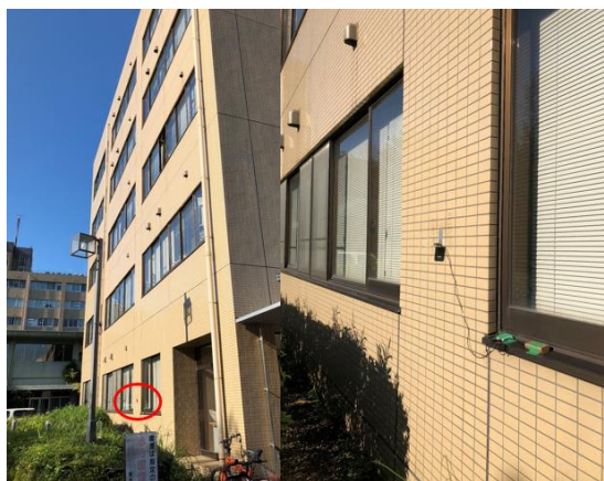
Fig. 10. Installation Status (southwest)
