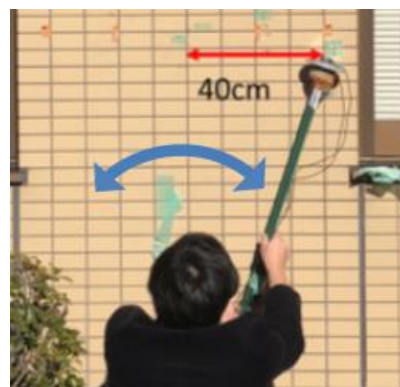
Fig. 26. Installation Status (southwest)
