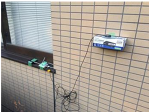
Fig. 7. Installation status (SW)
