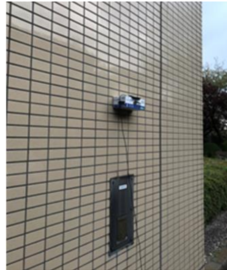
Fig. 9. Installation status (NW)
